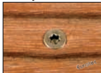
Pilot-drilling + Terrassotec screw
