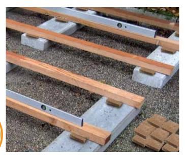
The cork pad spacers are laid between the deck substructure and the foundation/subsurface (self-adhesive on one side) and thus form a gap that aids constructive timber protection. The cork pad spacers are available in three sizes. These are 3 mm, 6 mm and 10 mm thickness/height (see Fig.). In addition to the advantages already mentioned, useful side effects of using the spacer include the option to adjust the height of the substructure and that the loads are distributed evenly.
