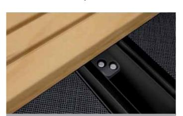
Hidden fastening using a deck glider on a Black Edition EVO aluminium system profile
