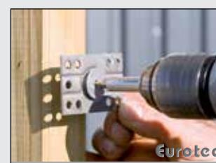
Screw the interwoven fence fitting with an interwoven fence screw at the head to the fence element. We recommend at least two fittings per side, ie 4 fittings for each fence element
