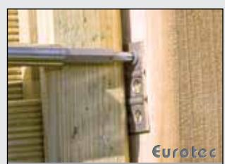
Now fasten the fence panel with the fitting to the wooden post. We recommend using 4 Clickyfix screws per fitting
